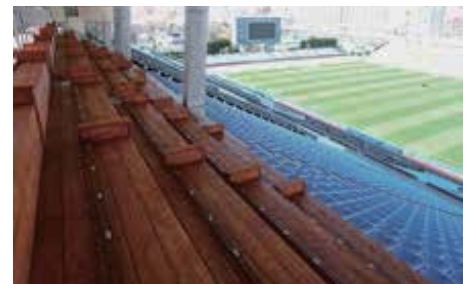
Benches of Maxelum and partly Koshii Super Thermo at the Kincho Stadium in Osaka
