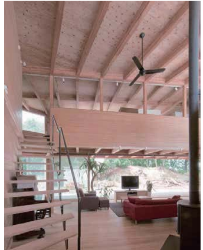
By using Nedanon, you can omit both horizontal braces and floor joists, which will simplify the construction process and increase the degree of designing freedom.
