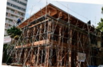
Figure 2. IBST wooden model construction. In parallel with this project, we are promoting industry-academia collaboration with the Hanoi University of Civil Engineering. This study is a joint research project on the production and use of wood and their strength characteristics.
